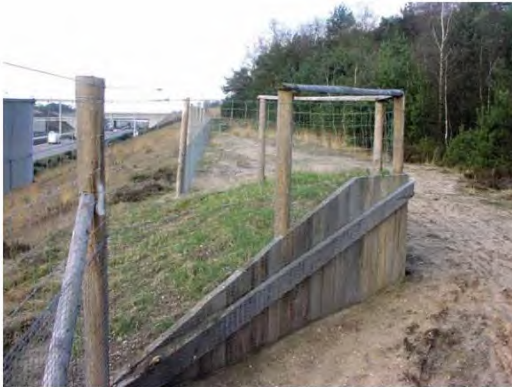
Figure F4: Large mammal exclusion fence made of metal wire and wooden poles (© T. Clevenger via Clevenger & Huijser, 2011). This photo shows an escape ramp (jump-out) for wildlife that get trapped inside the right-of-way. Note that this gauge of wire is not effective for excluding small animals, and metal posts are recommended over wood.
