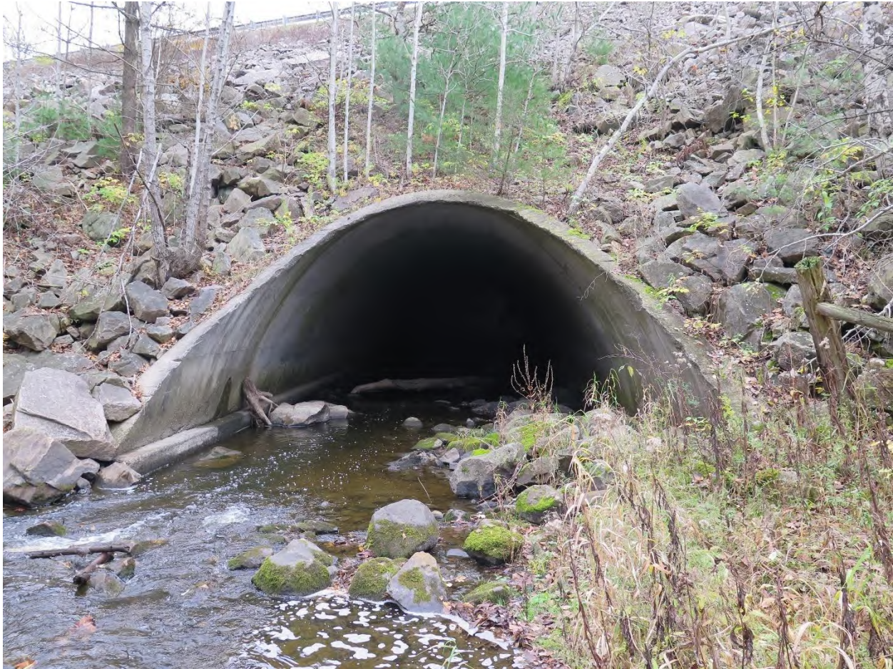
Figure 25: Photo of Jones Creek underpass at Highway 401.
