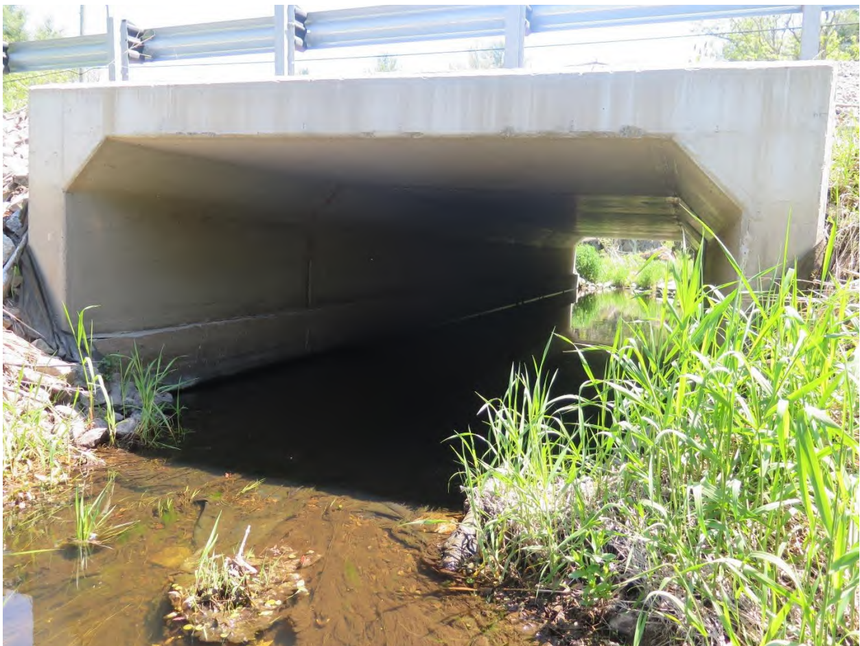
Figure 20: Photo of box culvert on County Road 2 within the Rockport to Waterton pathway.
