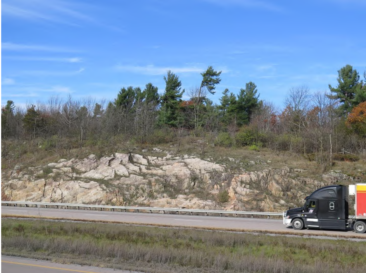
Figure 15: Photo of rock cuts along Highway 401 at the proposed overpass location within the Landons Bay to Lansdowne pathway.
