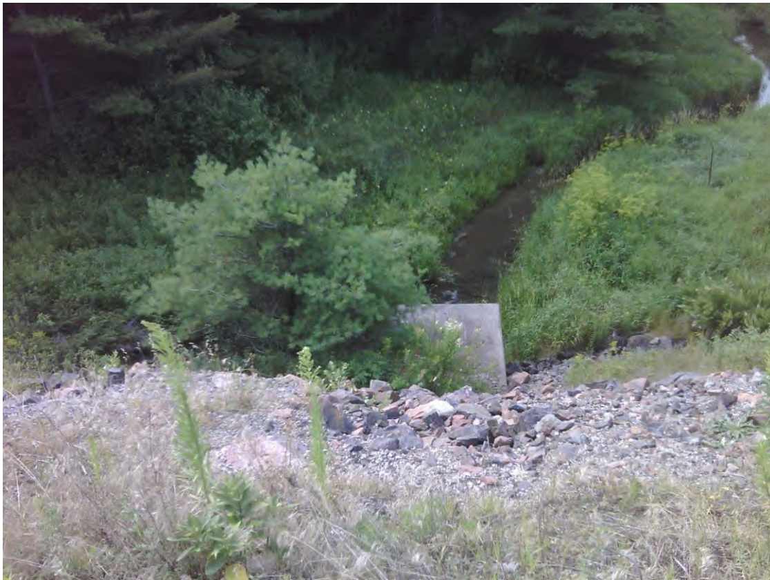
Figure 14: Photo of the existing box culvert at the Landons Bay Creek-Highway 401 crossing.
