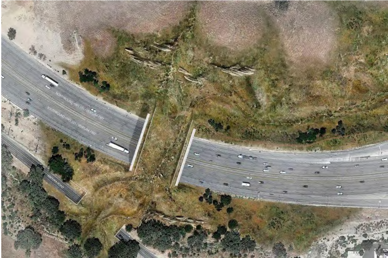
Figure D2: California's Wallis Annenberg Wildlife Crossing. Image source: https://www.newcivilengineer.com/latest/worlds-largest-wildlife-crossing-breaks-ground-in-california-22-04-2022/
