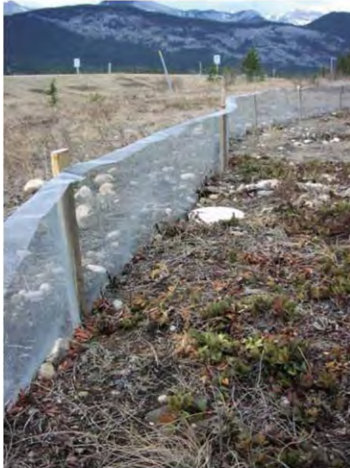
Figure F3: Reptile and amphibian fence with overhang, made of hardwire mesh and wooden stakes (© T. Clevenger via Clevenger & Huijser, 2011).
