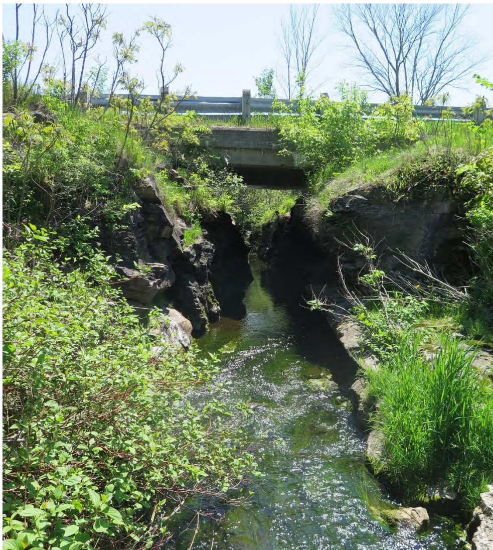
Figure 22: Photo of the bridge on County Road 2 that crosses a tributary of LaRue Creek.
