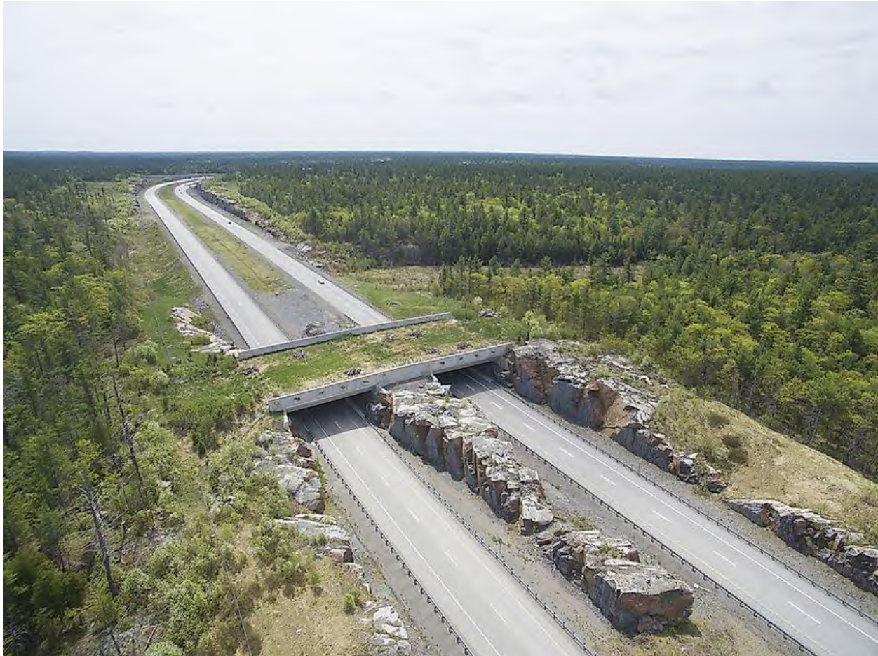
Figure D3: Wildlife overpass built on rock cuts. Image source: https://www.worldatlas.com/articles/what-is-a-wildlife-pathway.html
