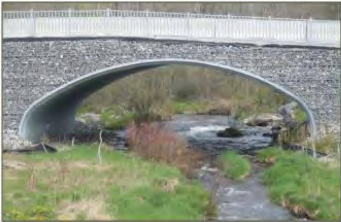
Figure E1: Wildlife underpass (arched tunnel) designed to incorporate a natural stream crossing and associated riparian area (© D. Seburn via OMNRF, 2016).
