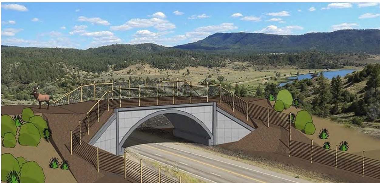
Figure D4: Example wildlife overpass design with fencing. Image source: https://coloradooutdoorsmag.com/2020/12/09/colorado-wildlife-crossing/
