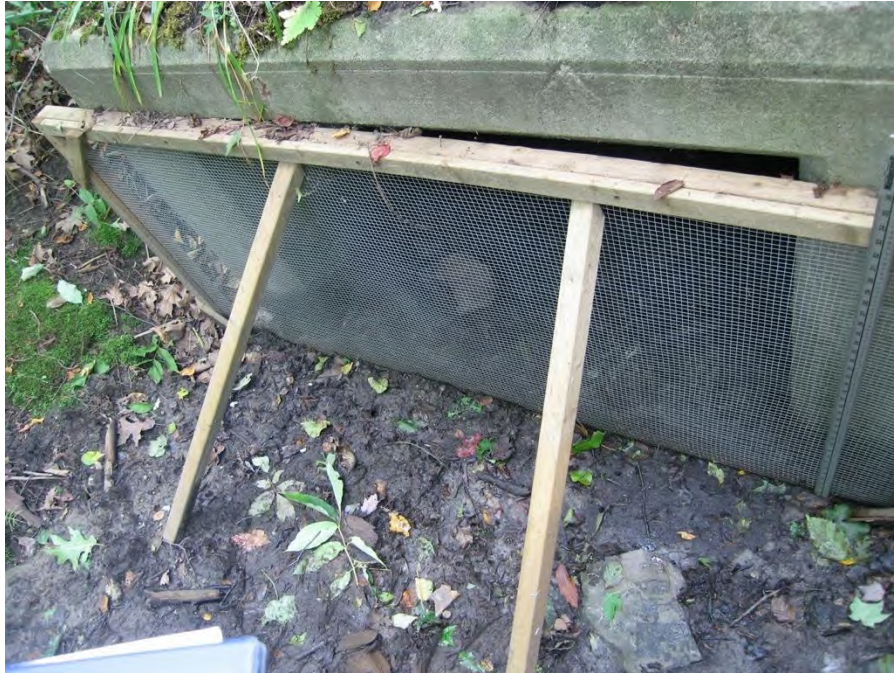
Figure B5: Grates were installed at six culverts along the Thousand Islands Parkway in 2009 and 2010 as part of a field experiment to evaluate the efficacy of culverts and roadside fencing in reducing vehicle-wildlife collisions. Results showed that culverts were effective for reducing road mortality but only when paired with fencing. Photo by R. Danby.
