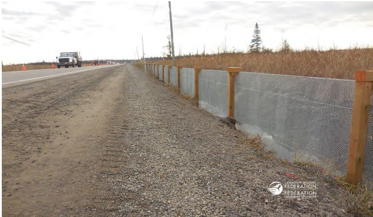
Figure F1: Roadside turtle fencing in Ottawa, made of hardwire mesh and wooden poles. Image source: https://blog.cwf-fcf.org/index.php/en/victory-for-eastern-ontarios-freshwater-turtles/
