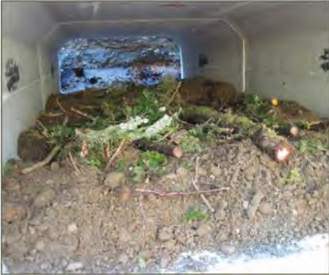
Figure E4: Wildlife underpass (box culvert) with soil and branches inside tunnel to increase microhabitat structure and complexity (© B. Beasley via OMNRF, 2016).
