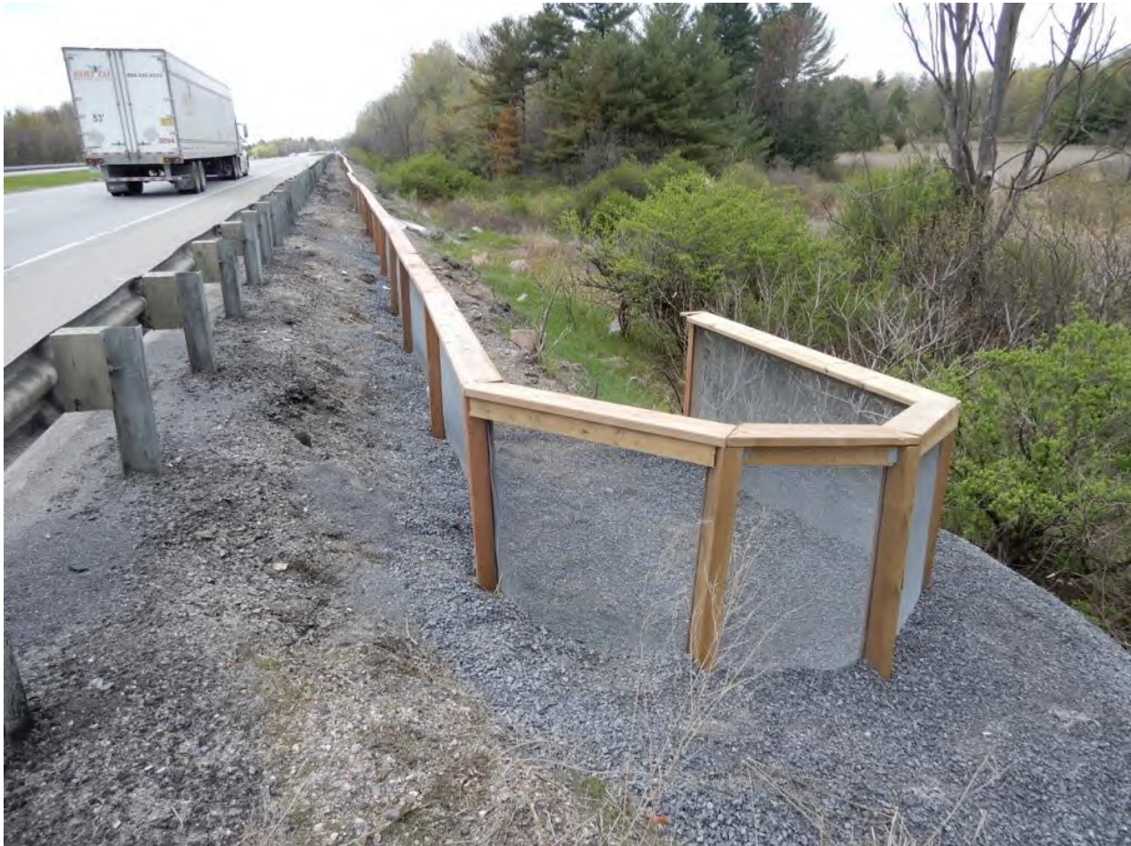
Figure B3: A section of fencing installed on Highway 401, intended to prevent entry of turtles onto the roadway and facilitate their use of existing drainage culverts for safe crossing. Photo by R. Danby.
